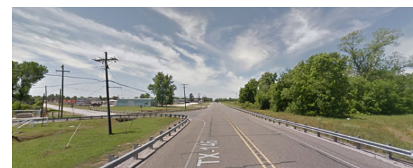
Figure 4.6 Minor Arterial - SH 146
